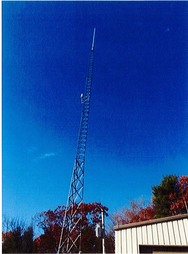
LEWISTON/AUBURN SITE – SHREDDER 100 FT. TOWER
