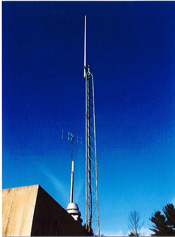
AUBURN SITE - HARDSCRABBLE 40 FT. TOWER
