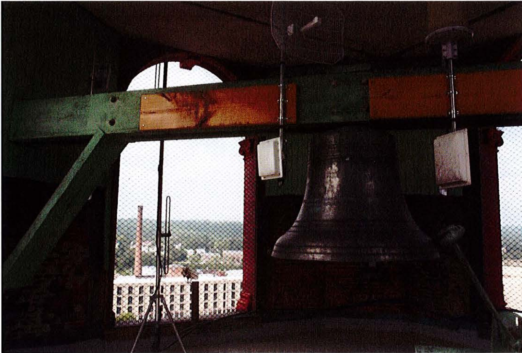
LEWISTON/AUBURN SITE - LEWISTON CITY HALL BELL TOWER (Photo provided by Lewiston-Auburn 911)
